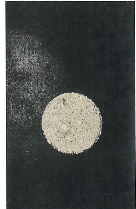
TH 2 Top of Asphalt Pavement Ø = 150 mm
